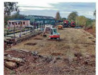
Construction of the Ironstone Railway Exhibition Centre commenced in October 2014.
